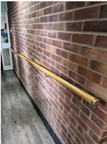
Handrails in the corridors
